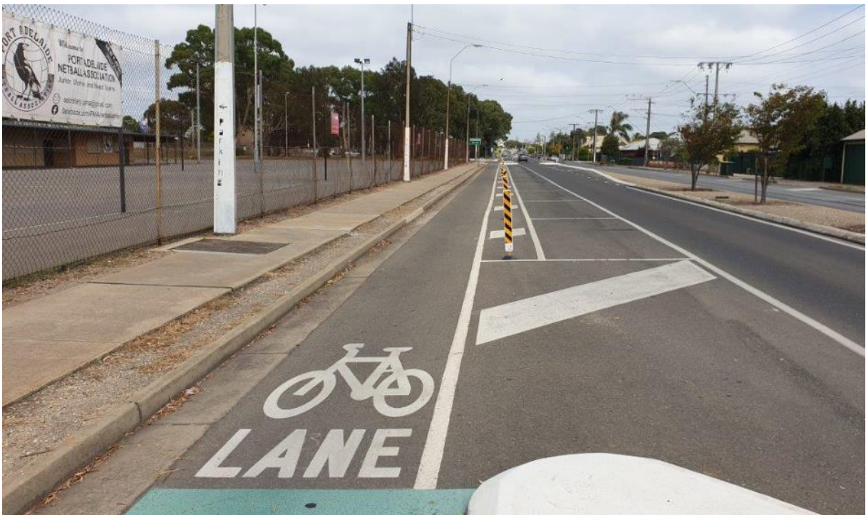
Figure 1: Separated cycle lanes installed by City of Port Adelaide Enfield council on Hart Street, Port Adelaide are an example of what 'good' looks like in relation to on-road cycle infrastructure and have created a much safer cycling environment.
