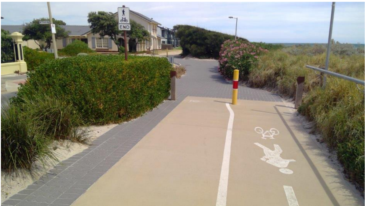
Figure 70: The end point of the existing northern path, looking south at Third Avenue, Semaphore Park
