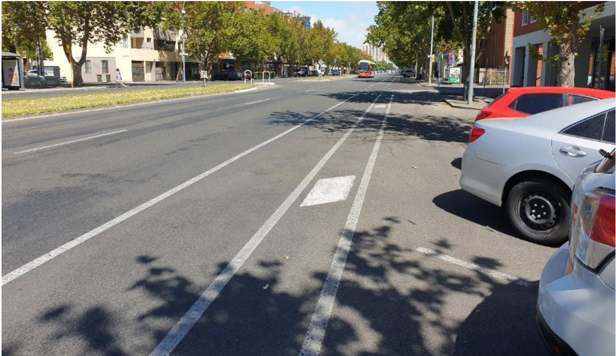
Figure 71: Current cycle lanes on Wakefield Street (pictured) and other east-west routes across Adelaide do not offer much protection to cyclists
