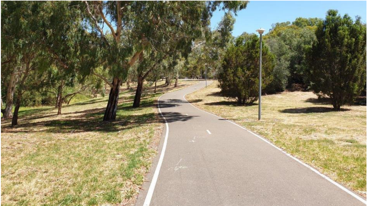
Figure 63: Many parts of the path are built to a high standard, with good width, line marking and provision of solar lighting
